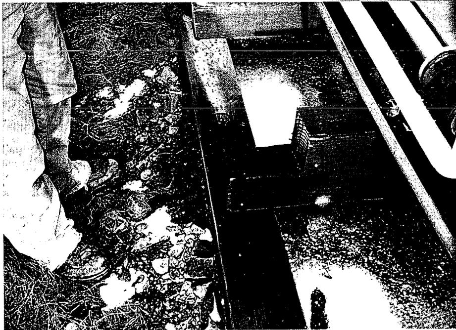
Photo 14: Tank Farm 7; Staining is visible on the timber comprising one side of the containment dike. This tank is supported by timbers spanning the dike. This tank farm was fenced but not locked.
