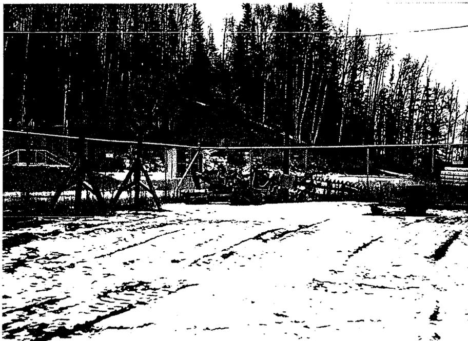
Photo 9: Tank Farm 5; The tanks from this tank farm have been moved to Tank Farm 6. The open area shown above is where the eight AVEC tanks were formerly located. The original pad has been covered with the gravel that comprised the former tank farm dike.
